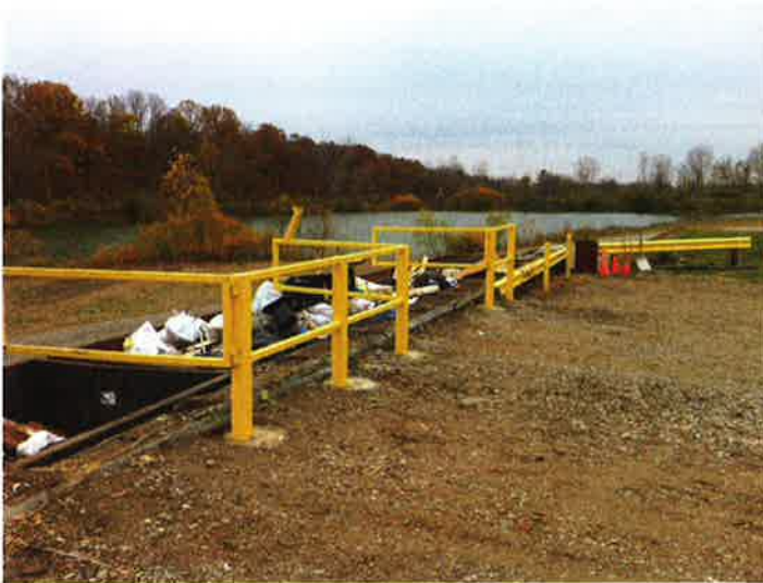
The first improvements to the LaGrange Convenience Center was safety railing.
